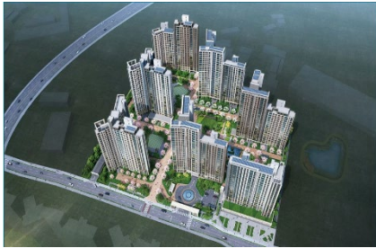
Bongdam Xi Lajeune (GS Construction)
